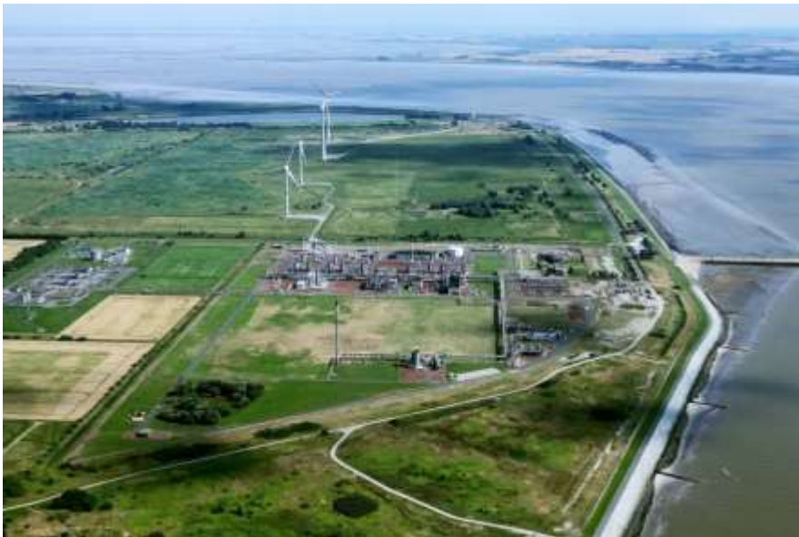
Port development project: „Rysumer Nacken“
